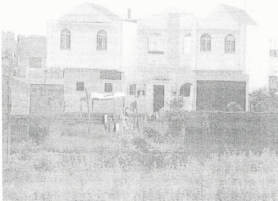
Habitat moderne Sangarébougou ACI
