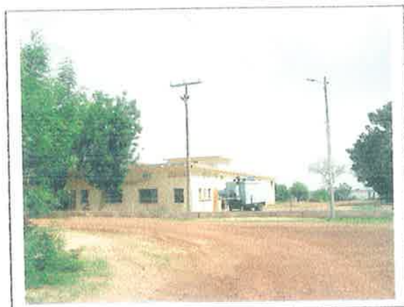
Station de Pompage
